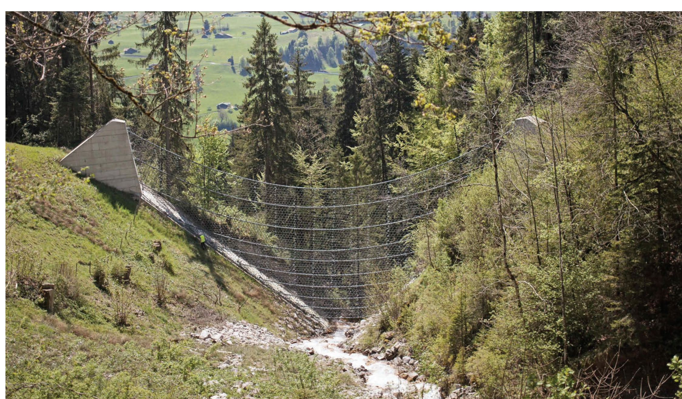
Special structure Hüpach/Switzerland with 40 m span and 10 m net height
