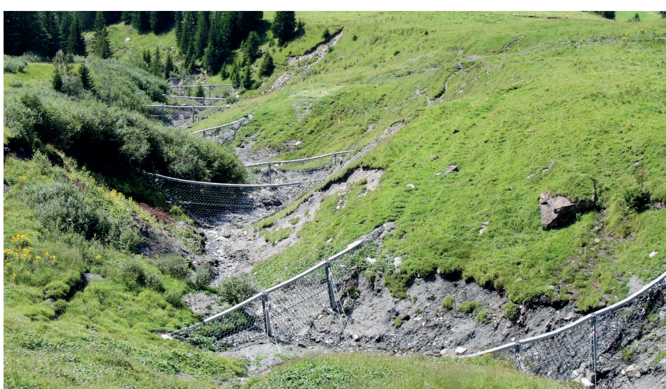
Multi-level debris flow barrier in Hasliberg/Switzerland
